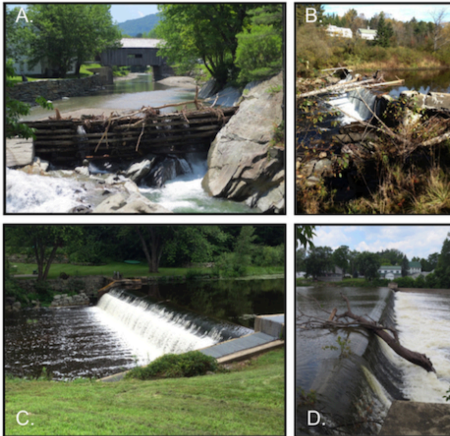
Fig. 1. Halted and stalled dam removals. (A) Warren Dam (B) East Burke Dam (C) Mill Pond Dam and (D) Swanton Dam.
